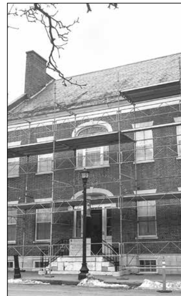
Photo contributed Robert Jenkins House under renovation.
